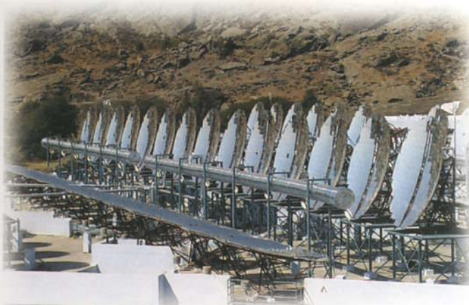
View of some of the parabolic converters at Shantivan
